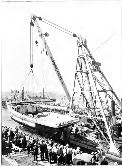
The above photograph shows the new fishing vessel City of San Francisco being launched into the waters of the Lagoon at Fishermen's Wharf, San Francisco, by the Haviside Derrick Barge No. 4. The vessel is 92 ft. long and weighs 110 tons. She was built at Fishermen's Wharf by the Genoa Boat Works for Beviavzua & Son, and is to be powered with Western-Enterprise diesel engines. Although the Haviside No. 4 has capacity for only 100 tons, the fishing boat was lowered without a scratch into the water, with a leeway of only a few inches on each side.
